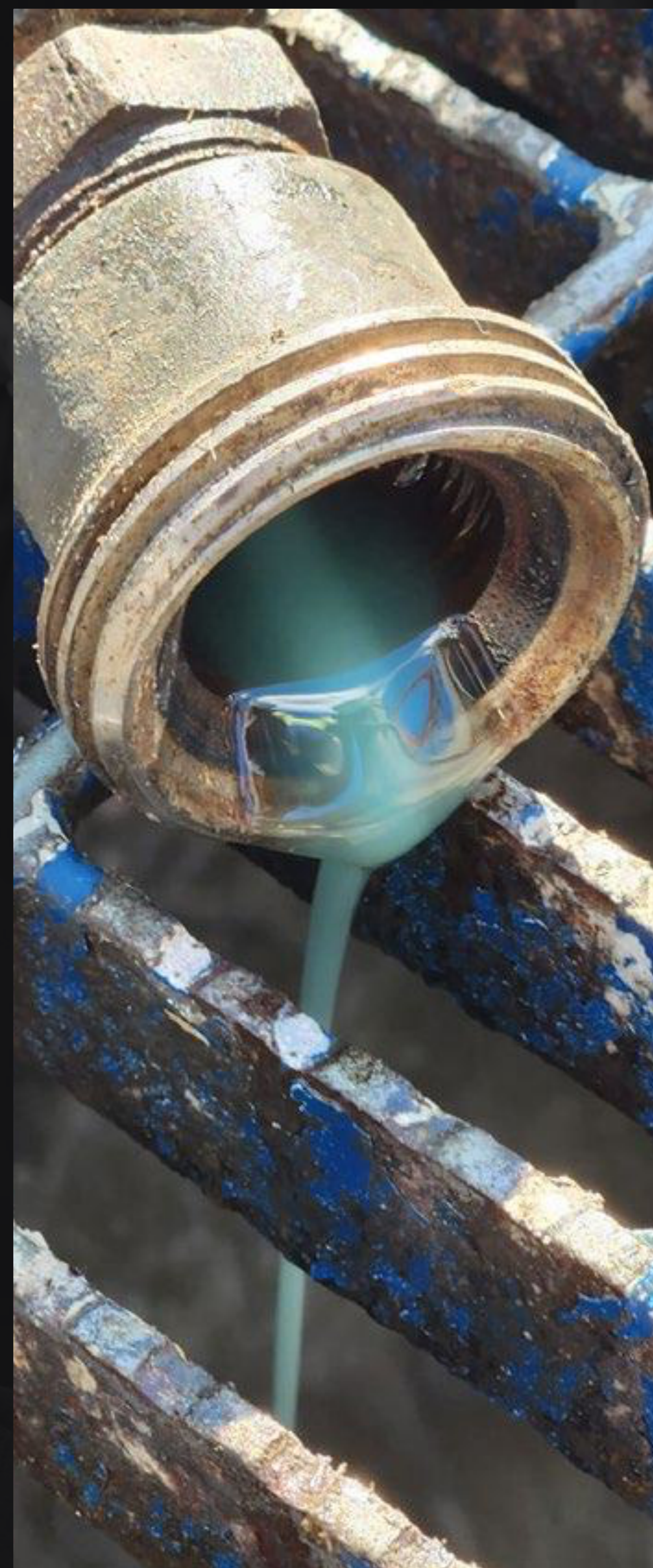
MDF Extendrill was added at <0.16% of the flow rate directly into the suction.
